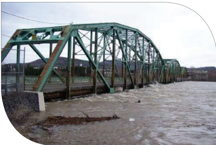
Flooded bridge on the St. John River in Maine. A major flood in 2008 was the highest flow measured at the U.S. Geological Survey St. John River at Fort Kent, Maine station (01014000), based on a record going back to the 1920s. Photograph by the U.S. Geological Survey.
